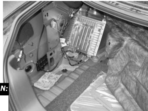
In some vehicles, the factory CD changer connections are made in the trunk.
